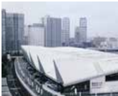
Water saving through utilization of roof rainwater
